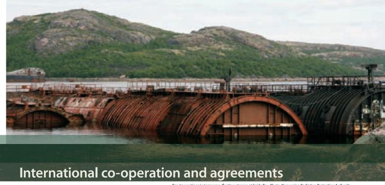
Reactor sections in temporary floating storage at Saida Bay. Photo: Norwegian Radiation Protection Authority.
