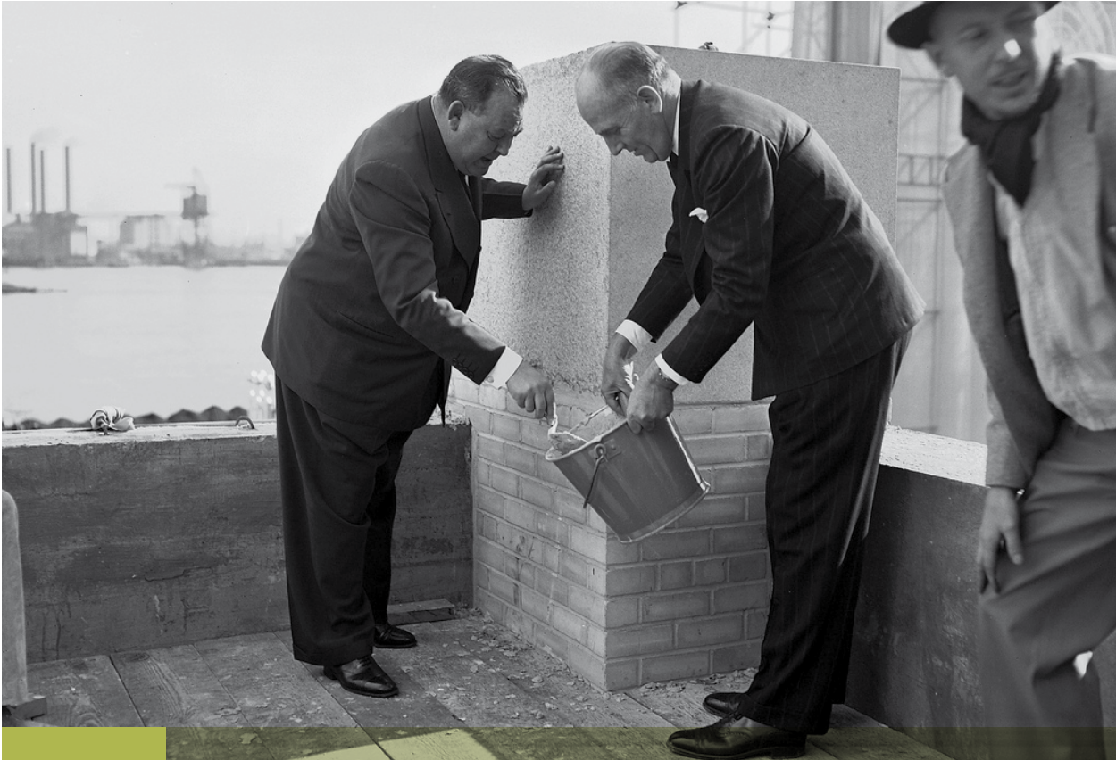
Trygve Lie, the first Secretary-General of the United Nations laying down the cornerstone of the new permanent headquarters of the UN on 24 October 1948, together with Wallace K. Harrison, Chief Architect of the Building. (Photo; UN.N.Y)
