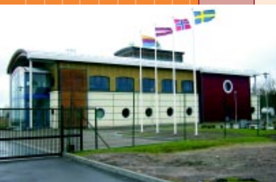
The Baltic States Diving Training Center (BSDTC) in Liepaja opened in 2001. Ships' and mine clearance divers trained here are part of the Baltic Mine Clearing Squadron (BALTRON).
