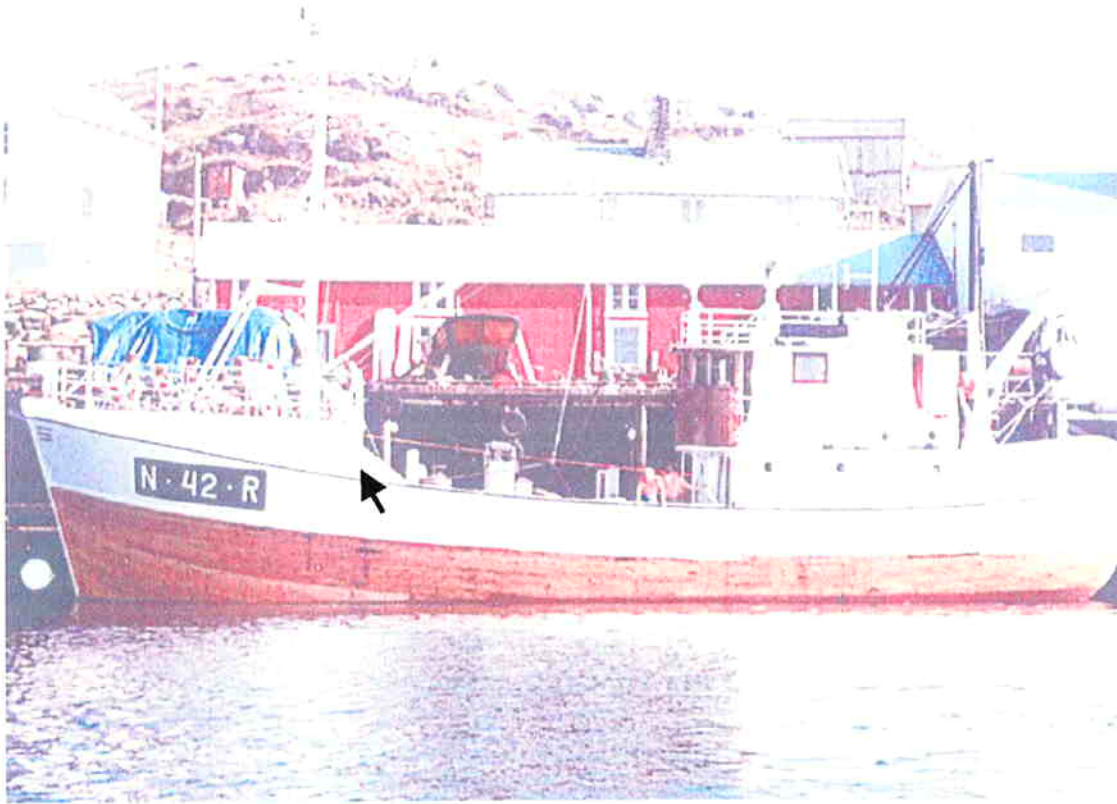
(Small) Hole in port side ( aft of forecabin bulkhead) approximate position indicated by black arrow
