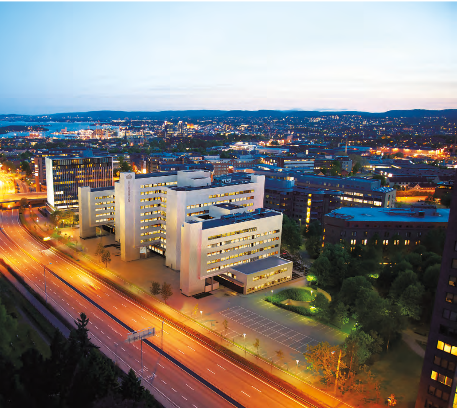
FREDRIK SELMERS VEI 4: The offices of the Directorate of Taxes are being fully renovated to the passive house standard. Photo: Entra Eiendom
