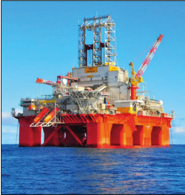
Figure 3.11 Winterised drilling rig. Transocean Barents.
