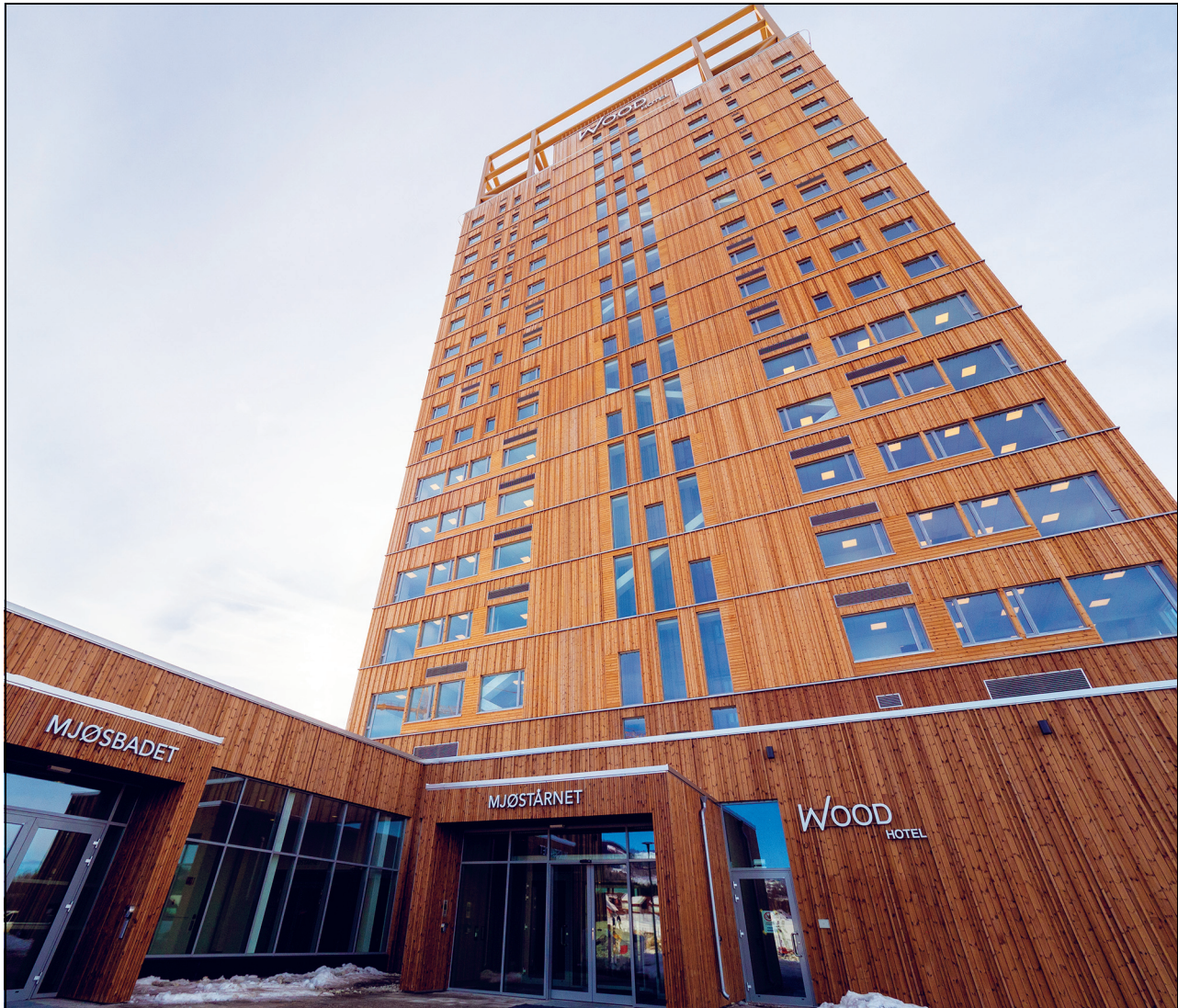
Figure 7.1 Mjøstårnet (the Mjøsa tower) is the world's tallest wooden building, and stores carbon equivalent to 3 000 tonnes of CO 2 .
