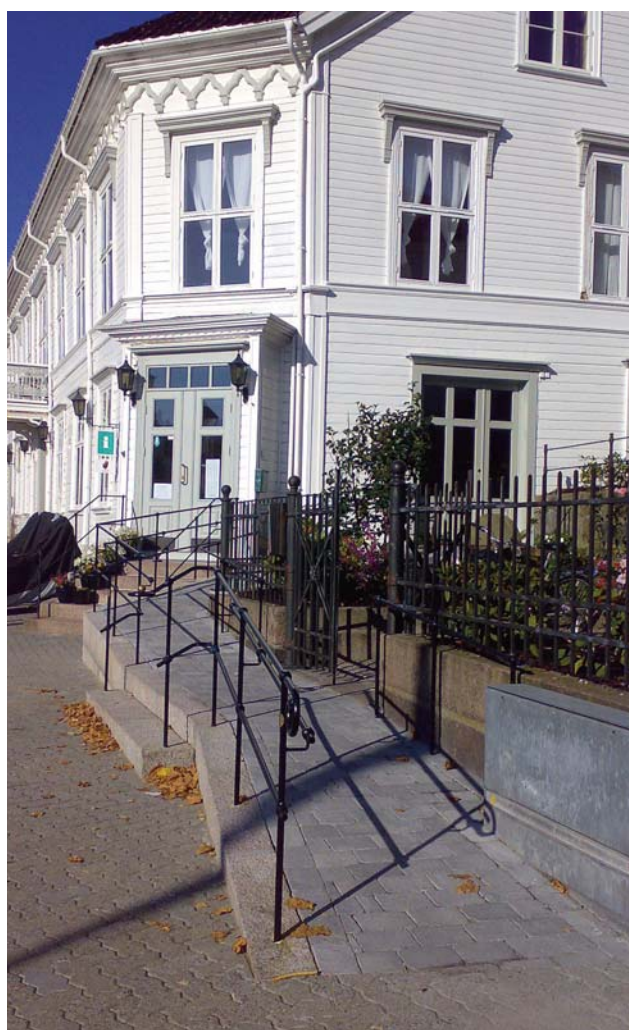
The new tourist information office in Risør. A new entrance has been built in an old window opening and a ramp installed as a new part of an existing green park. Photo: Risør municipality
