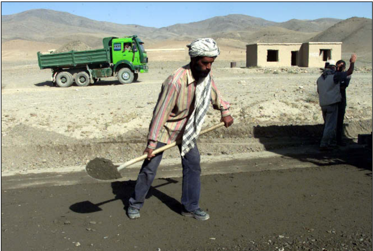
Figure 9.1 Building a road in Afghanistan
