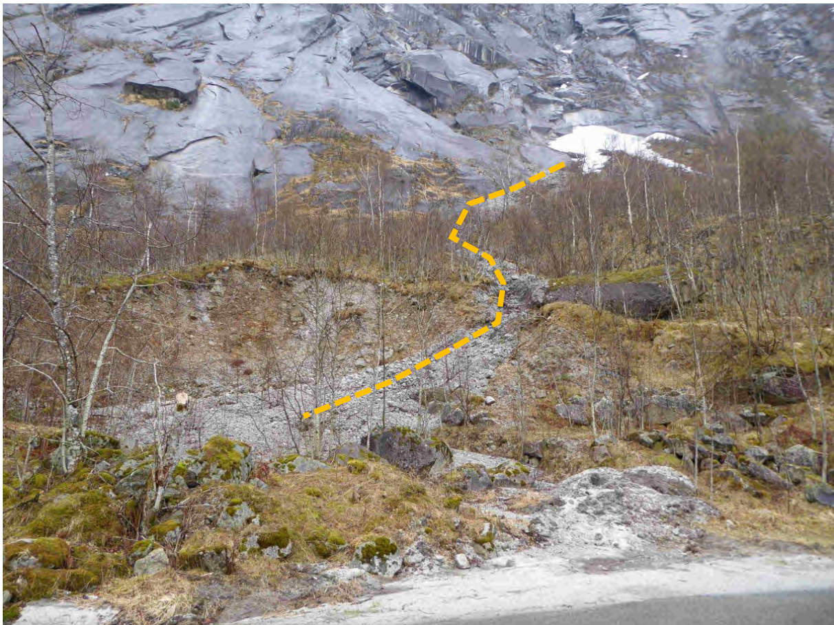
Figure 10: Recent debris flow consisting of gravel and rock fragments that have reached the road at the southern margin of the assessed converter site area.
