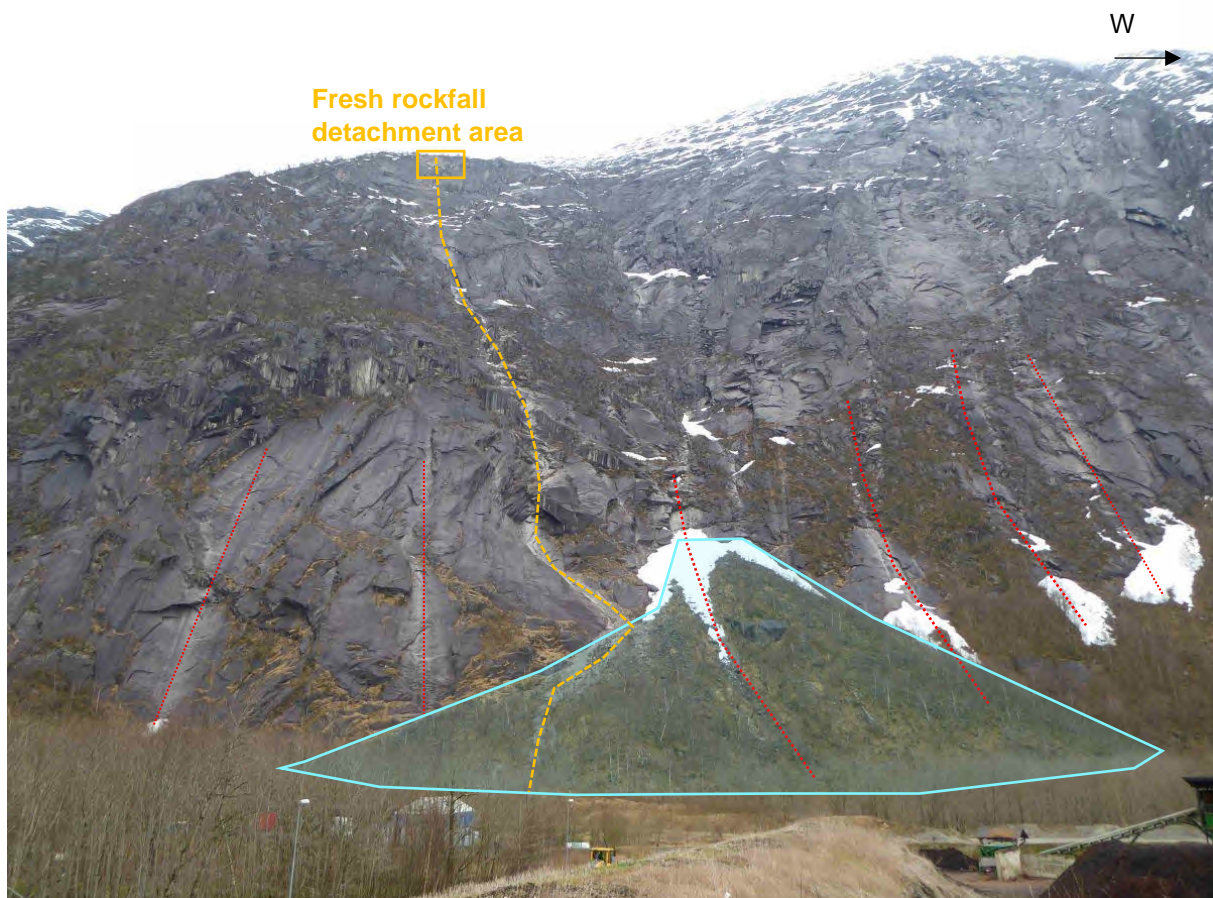
Figure 6: Photo that show southern part of converter site area and the southern mountainside. Talus has blue hatch. Registered paths for recent events are marked with red, orange line show recent rockfall/debris flow that released around 720 m.a.s.l and extended to the local road at the southern margin of the converter site.
