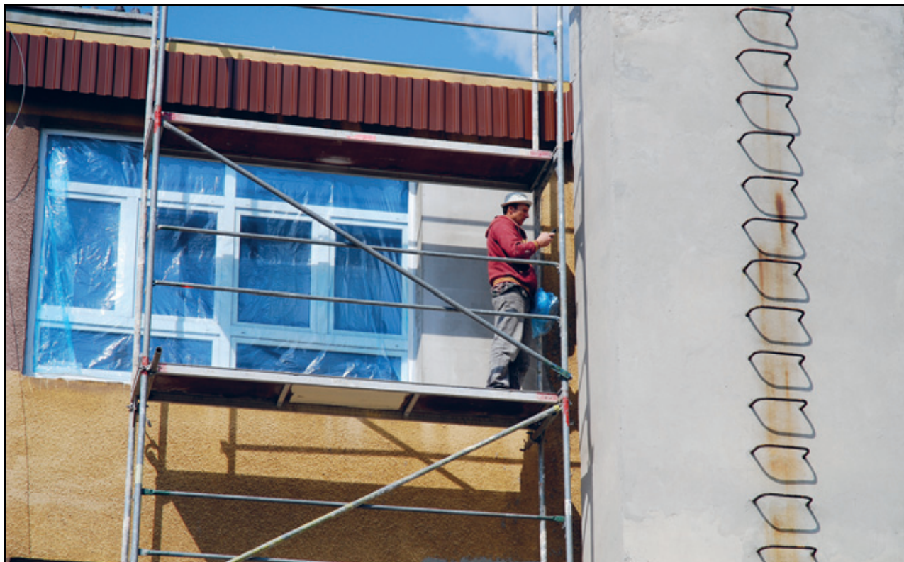
Figure 3.1 Improving energy efficiency in buildings is one of the most effective means of reducing greenhouse gas emissions. This building in Busko, Poland, is one of seven school buildings that have been reinsulated and given new windows and doors.
