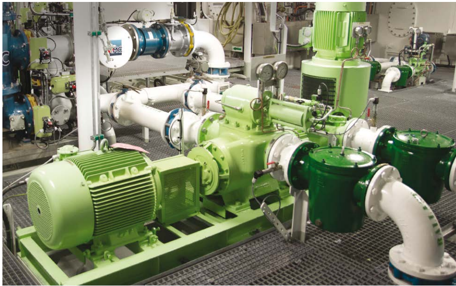
Cleaning system for ballast water installed on board Esvagt Faraday. Photo: Gunnar Larsen
